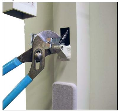
**12** Crimp bracket onto cable as shown below.
