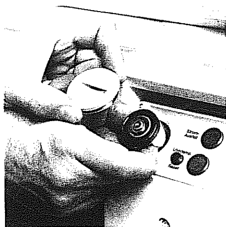
Fig. 44 Replacing battery for power-failure alarm
